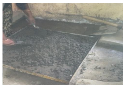
Fig. 6 Preparation of Concrete
