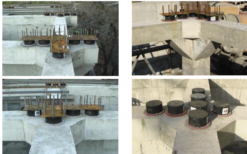
Figure 3. Examples on installation of clusters with different numbers of rubber bearings
