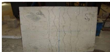
(a) Slab S1; ordinary concrete without steel
