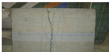
(e) Slab S5; HSCC with steel fibers (0.75%)
