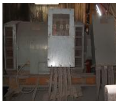
Fig. 3. 937 kW Unregulated motor with shaft mounted fan cooling arrangement.
