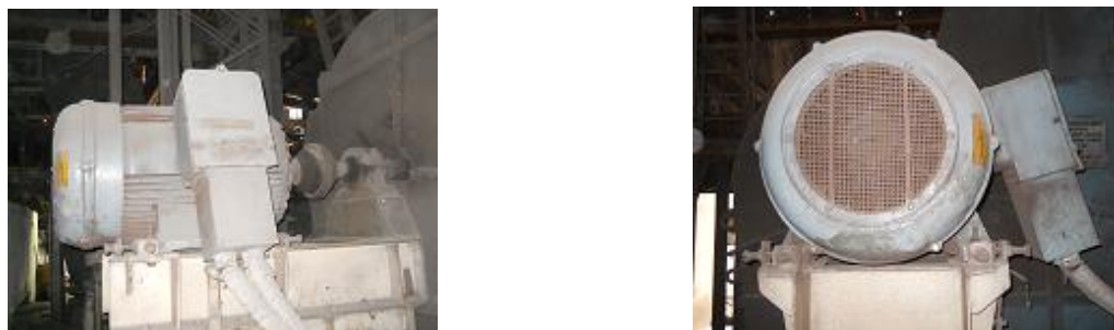
Fig. 1. Unregulated motor with shaft mounted fan cooling arrangement.
