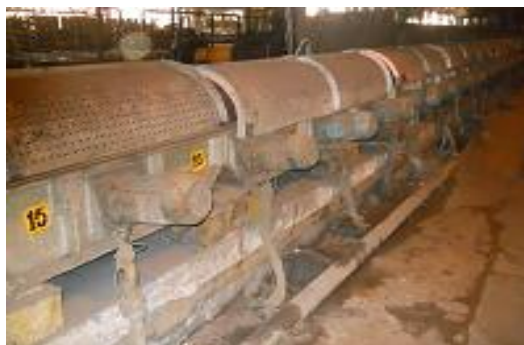
Fig. 5. Regulated motor with fan on shaft for cooling
