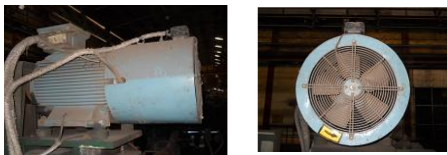
Fig. 4. Regulated motor with external fan cooling arrangement.
