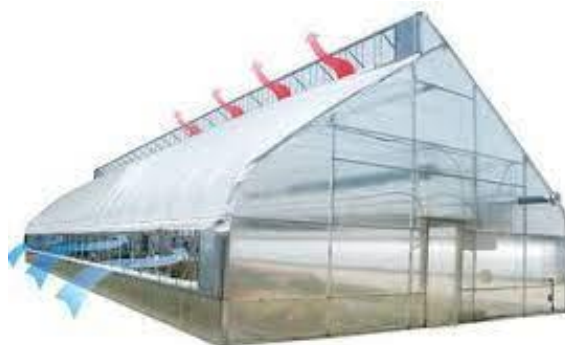
Figure 1.3. Ventilation in greenhouses.
