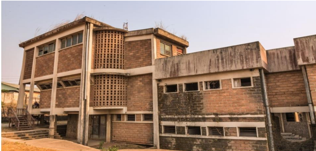
Figure 6. New Culture Studio – An example of Institutional Building in Sustainable Architecture
