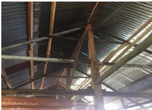
Fig 4. Roof truss seen from inside the house
