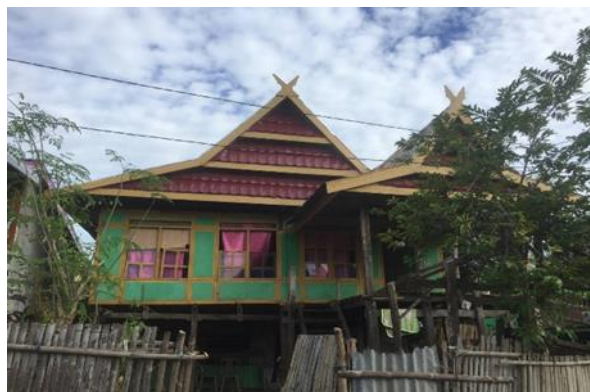
Fig 3. Outer roof view
