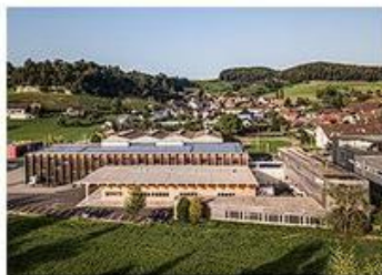
Precedent study 1: Schaerholzbau Grossdietwil Furniture Factory
